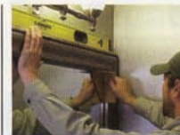
Adhere the placement corners to the mirror, then install the frame using the adhesive strips on the rear.
