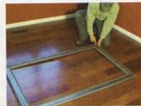
Tap in the plastic connectors and remove the excess glue.
