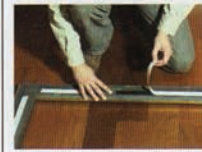
Adhere the placement corners to the mirror, then install the frame using the adhesive strips on the rear.
